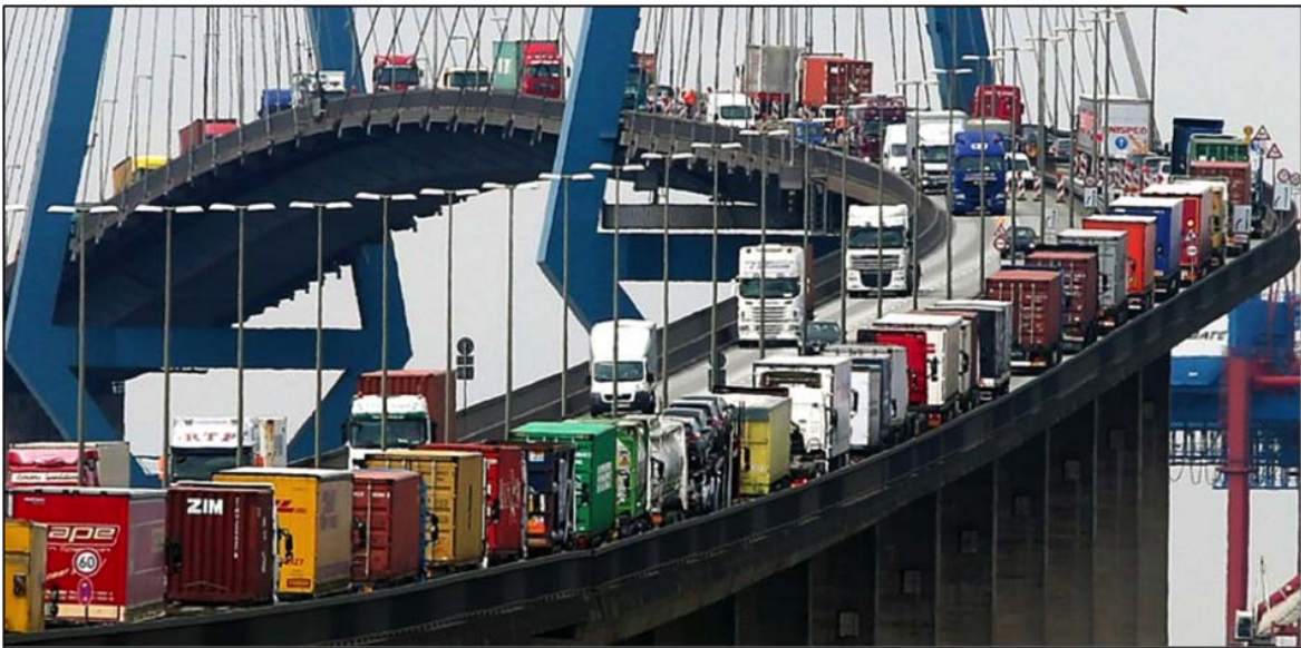
Fig. 1: Typical view on Hamburg's Koehlbrand Bridge linking the eastern and western part of the port
