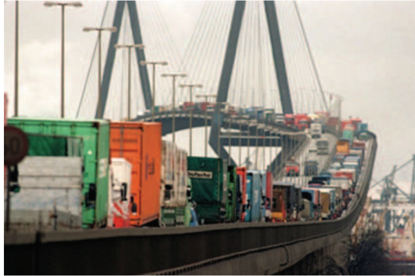
Fig. 20.4 Typical view on Hamburg's Köhlbrand bridge linking the port's eastern and western part (German Press Agency)
