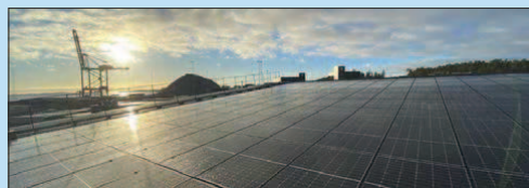
A section of the warehouse roof at Stockholm Norvik Port
